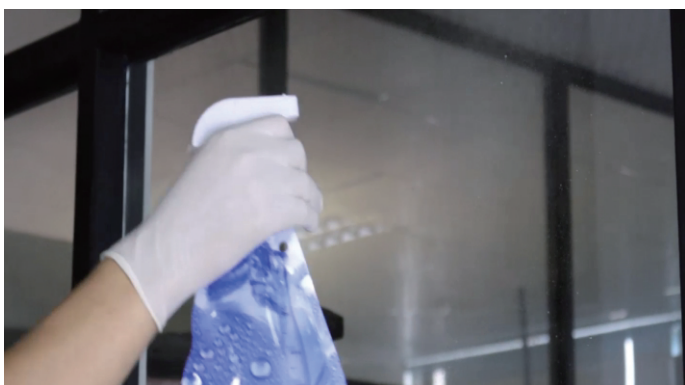
3. Clean the glass before installation
