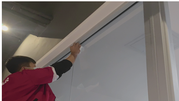
4. Dry glass before installation
